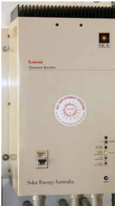
This type of inverter is hard-wired into the RV's mains wiring system..
